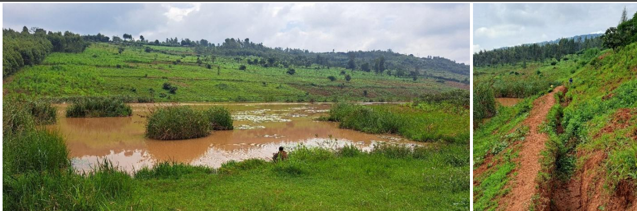
View of Bisinia Dam and the trench below the Musha mining activities
