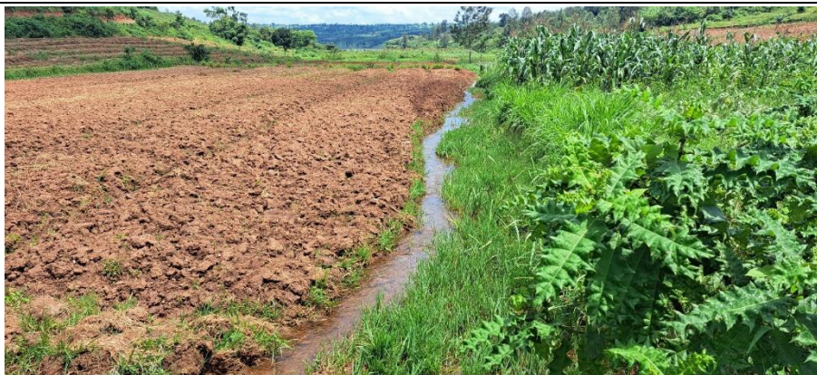
Main drainage channel within the system
