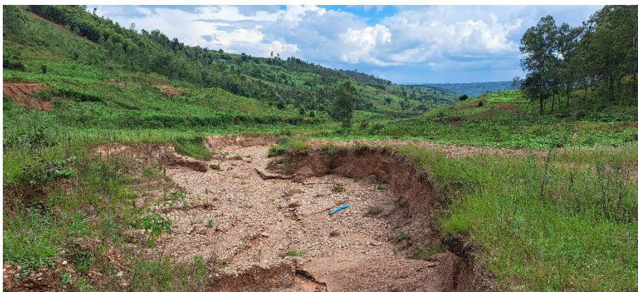
Figure 5-15 Gully erosion directly downstream of the Ntungwa Mine
