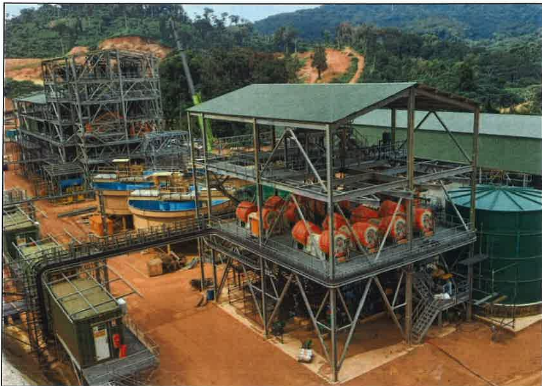
Image 1: Mpama South Tin Concentration Plant during construction
