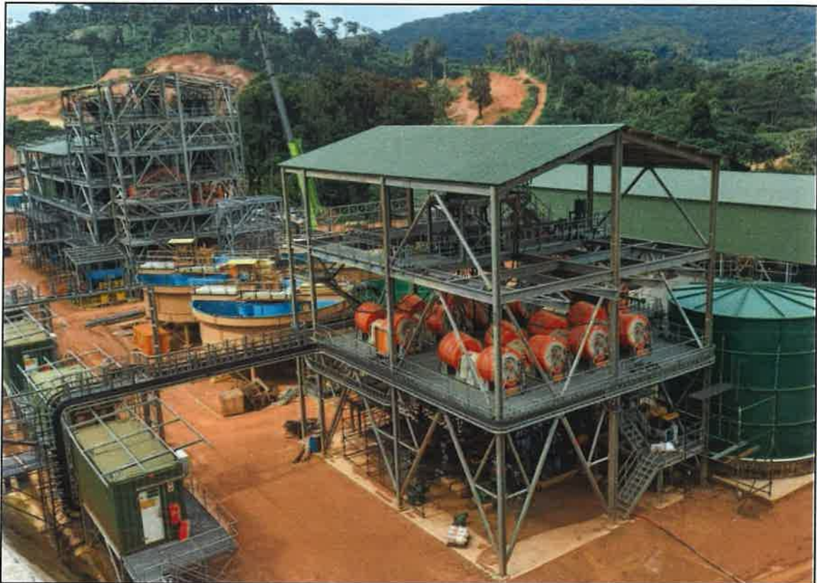
Image 1: Mpama South Tin Concentration Plant during construction
