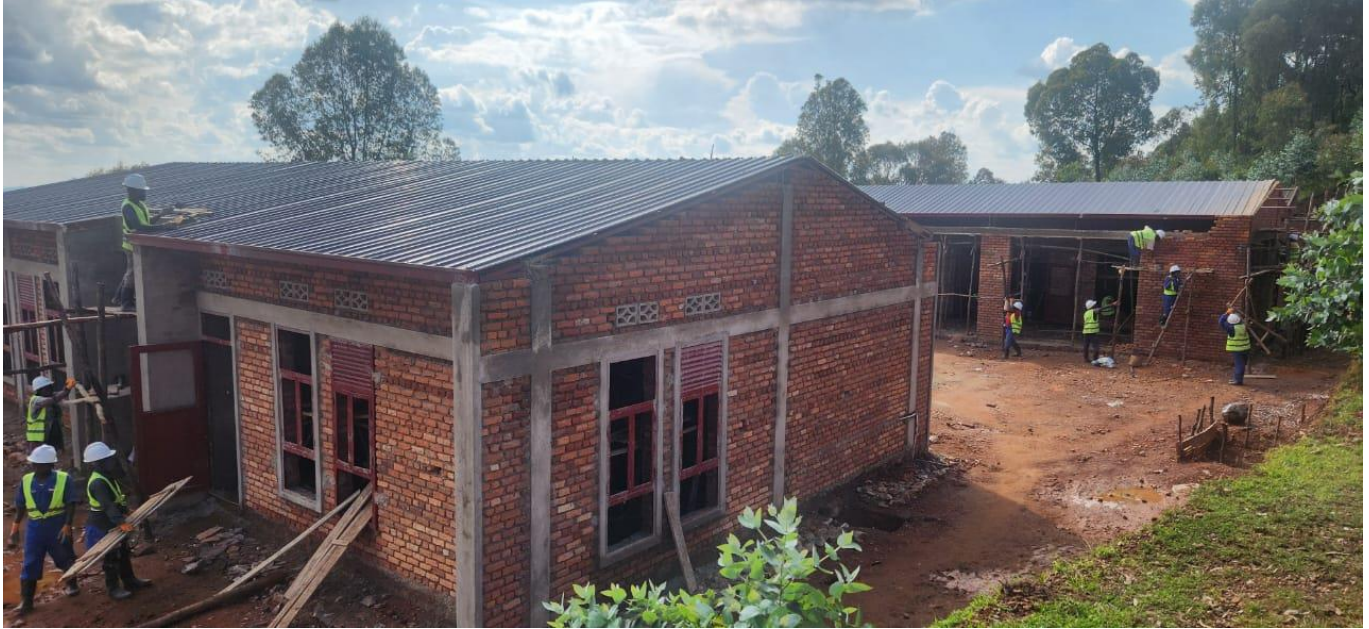
Figure 1: Roof covering with ironsheets completed
