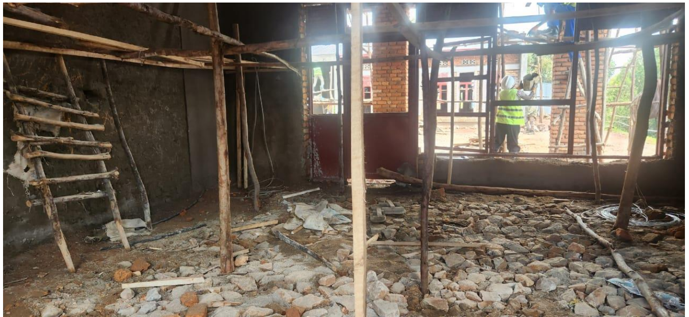
Figure 2: hardcore layer pavement
