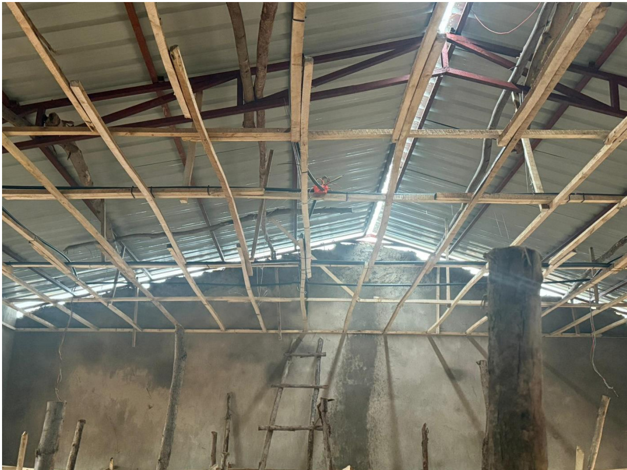
Figure 6: Electrical installation done
