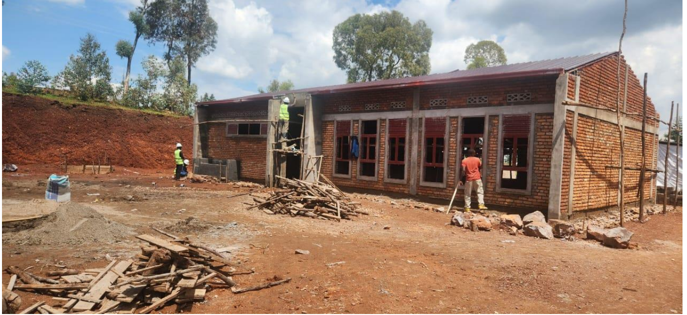
Figure 5: Sleeping area external wall finishing
