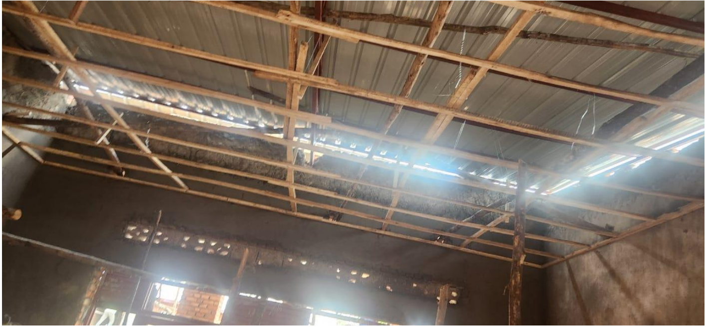
Figure 3: Timber for ceiling completed
