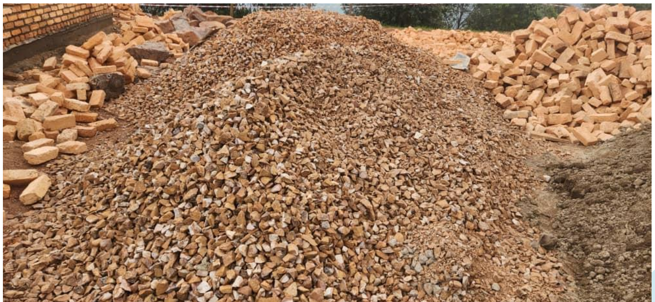
Figure 2: Gravel Materials for concrete works
