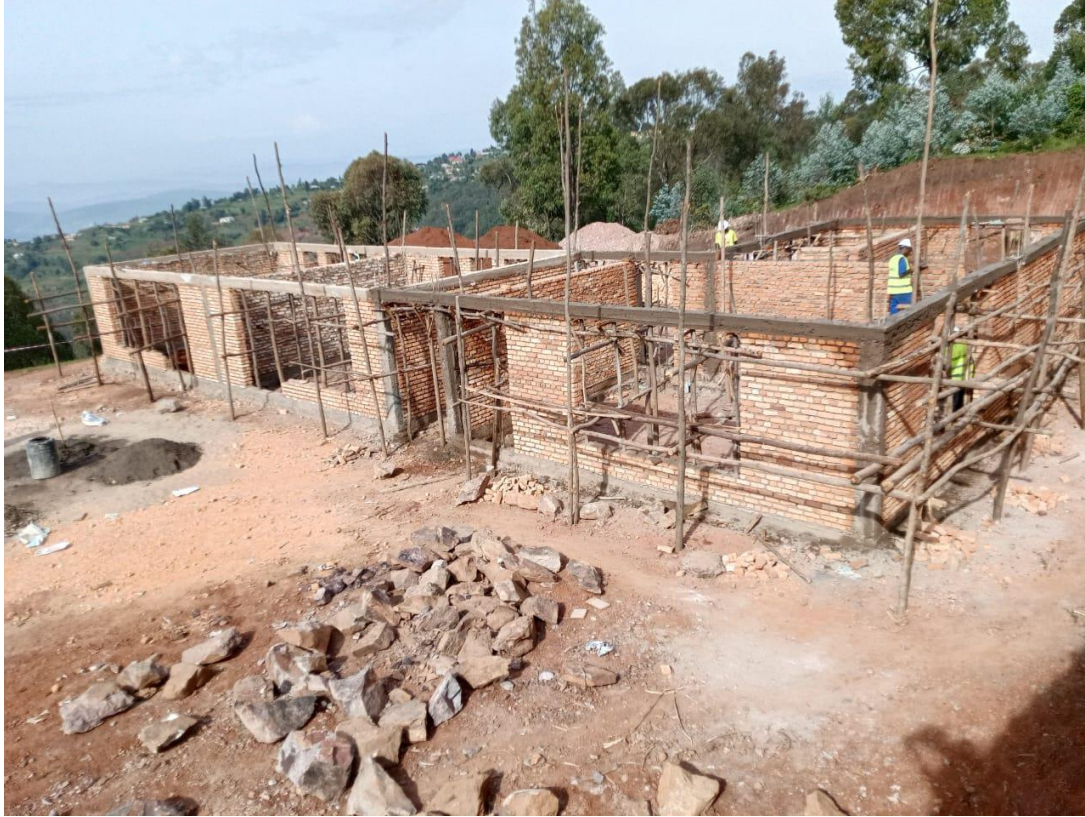
Figure 5: Works reach at lintel lever
