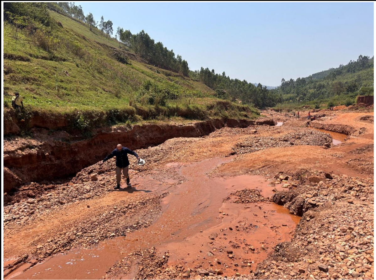
Photograph showing highly modified channel due to sand/aggregate mining.
