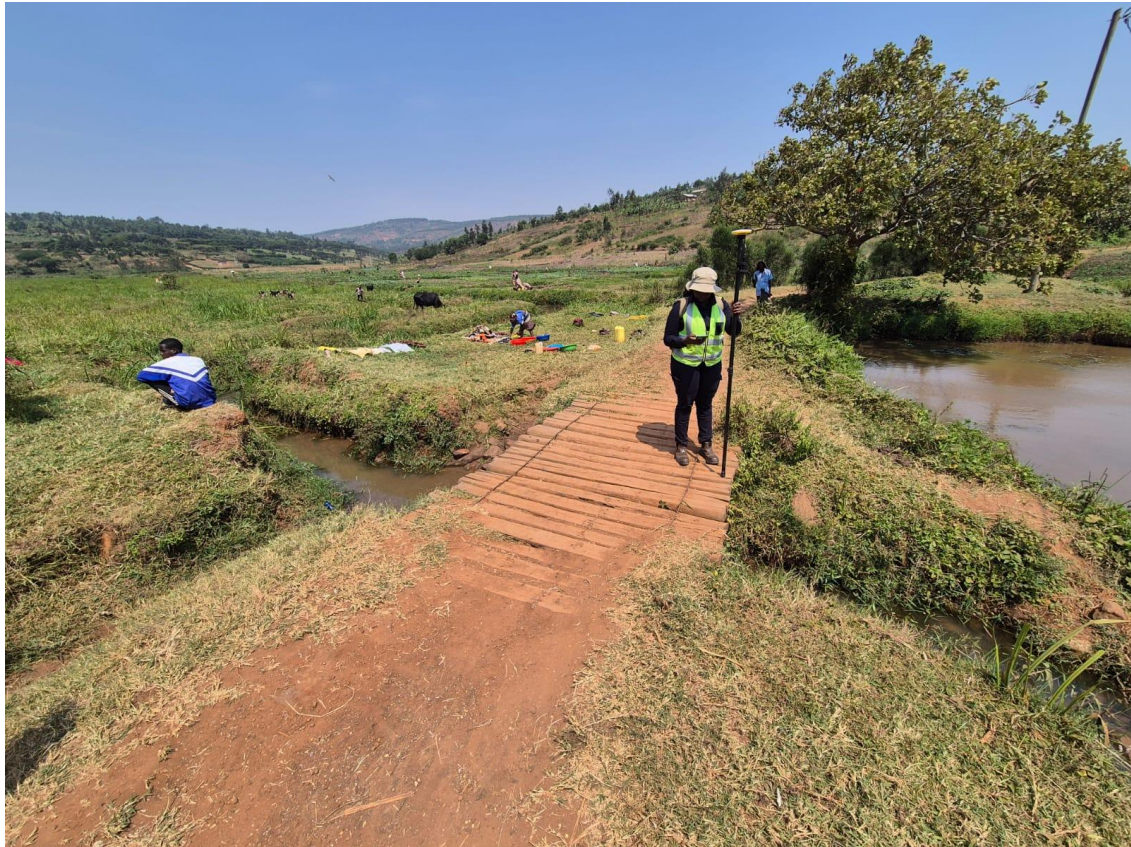
Photograph showing team member surveying pedestrian crossing erected over watercourse.
