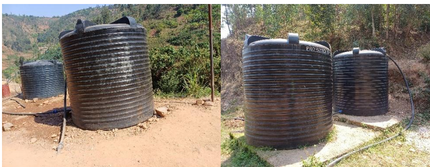
Tanks at Tunnel 11
