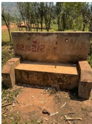
Water collection point
