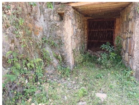
Locked entrance to Tunnel 7
