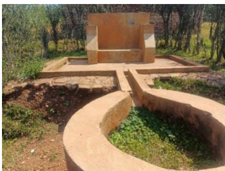
Water distribution point
