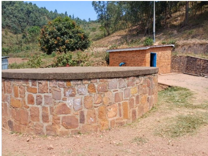
Tank and Pump at Musha Mine
