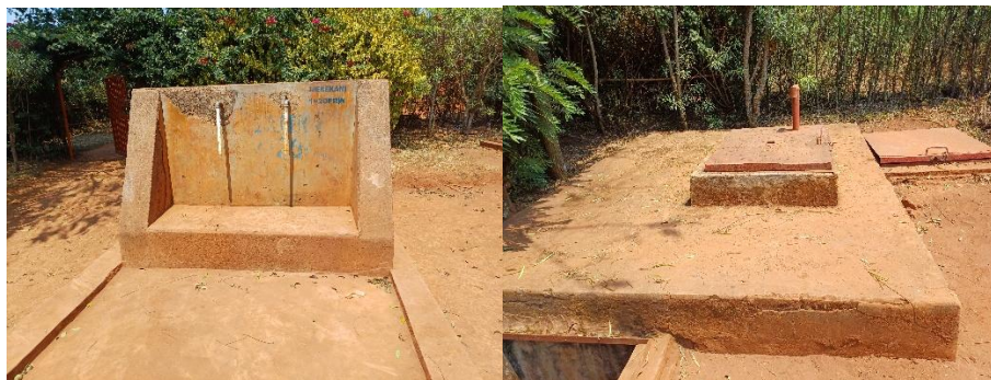
Water collection point
