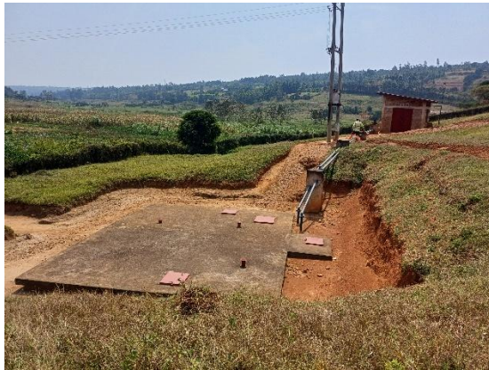
Tank at source and pumphouse
