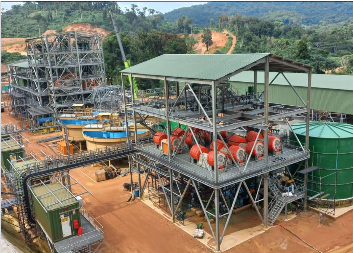
Image 1: Mpama South Tin Concentration Plant during construction
