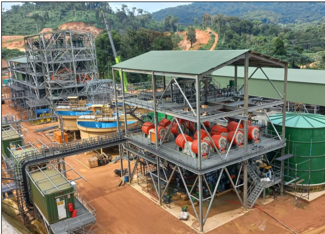
Image 1: Mpama South Tin Concentration Plant during construction
