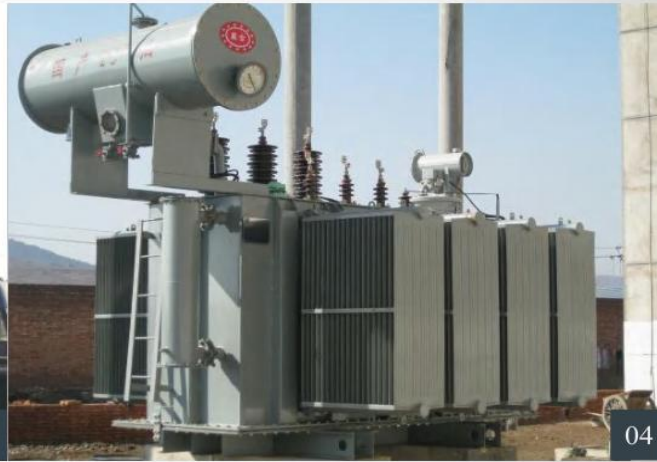
SZ11-10000/35 State Grid Songxian Manyu Substation Installation
