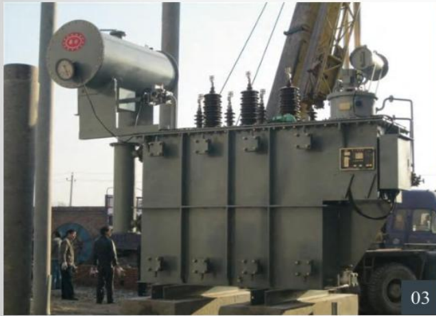
SZ11-10000/35 State Grid Songxian Manyu Substation Installation
